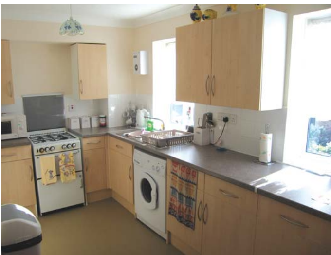
A new kitchen installed under Decent Homes.
